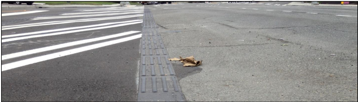
Tactile Crosswalk Installation at Rainier Ave S and 23rd Ave S
