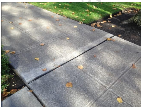
Beveling (or grinding) Sidewalk Uplift to Make Smooth Sidewalk Transition
