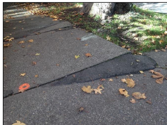
Asphalt Shims Applied to Make Smooth Sidewalk Sidewalk Transition
