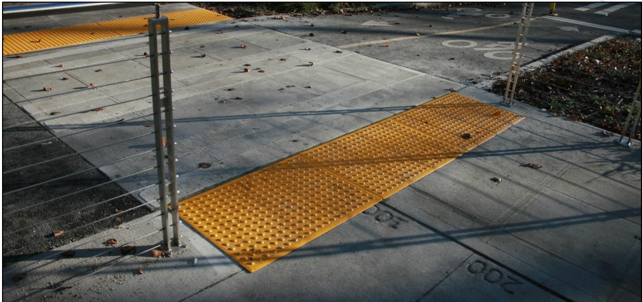
Detectable Warning Surface Installed at Broadway Streetcar Platforms
